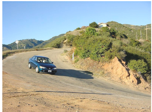
Figure 10. Hairpin bend on San Marcos Road. Average grade over 10 km is 8%, and separation on hairpins is 15-20 m.
