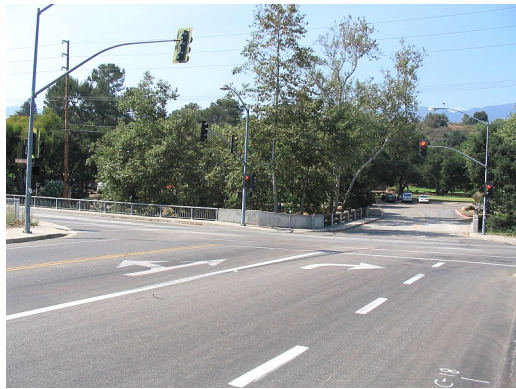
Figure 4. Turnpike at Cathedral Oaks, Santa Barbara (intersection A in Figure 5), looking north. No physical separation of lanes.
