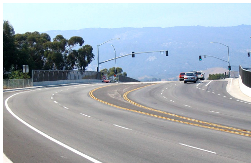
Figure 7. Fairview overpass: opposing traffic separated by double yellow line only.
