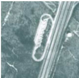
Figure 1. I-95 Dumfries, Virginia.
