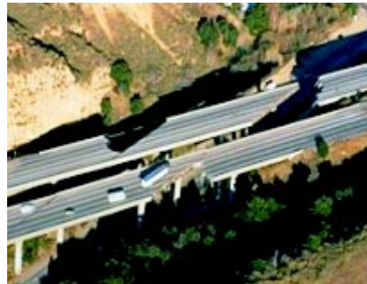
Figure 1. Earthquake damage to a bridge on the I-5 in Gavin Canyon.
